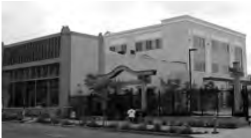
Jodo Shinshu Center in final stages of construction in Berkeley.
